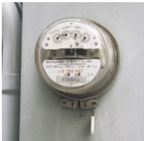
Figure 2 Readings from electrical meters are used to calculate the amount of energy used.
