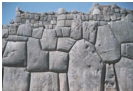
Figure 5 Tight-fitting stones of a large Inca wall near Cuzco, Peru
