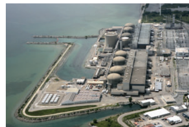
Figure 3 The Pickering, Ontario, nuclear power plant is built near an adequate water supply (to keep the fuel rods cool).
